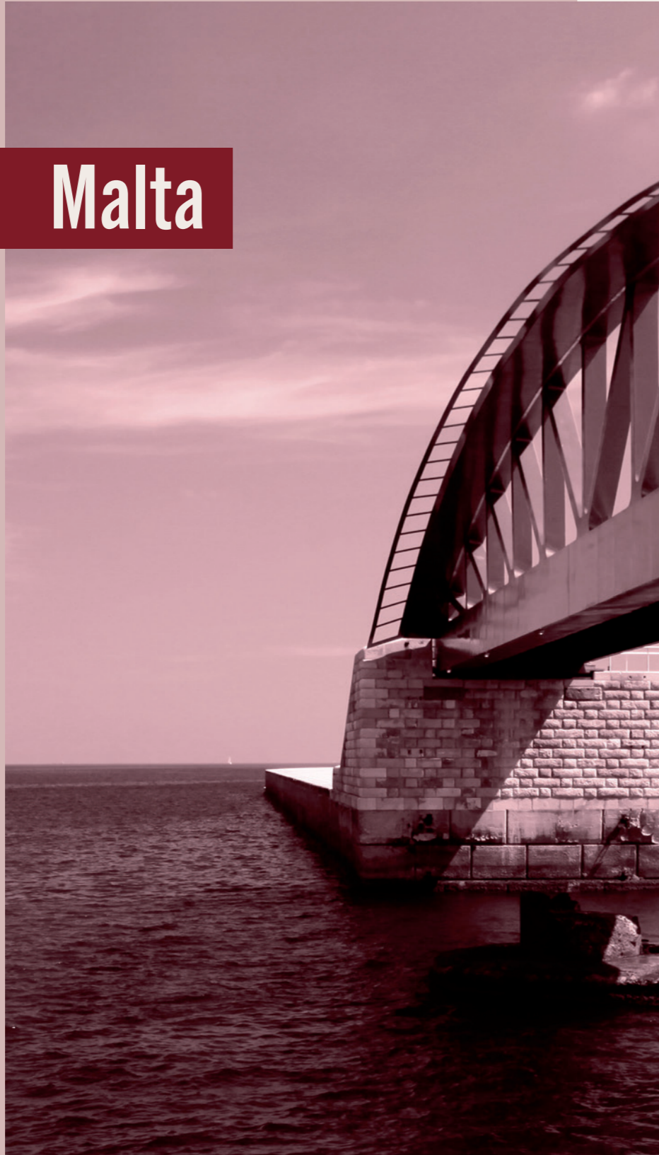
The Breakwater bridge, La Valletta
