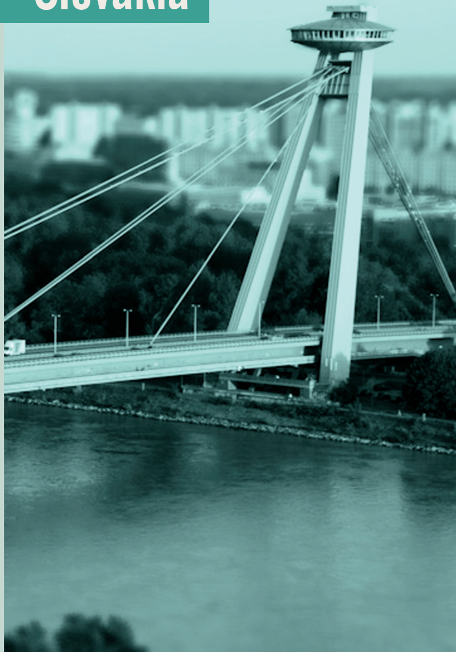
New bridge, Bratislava
