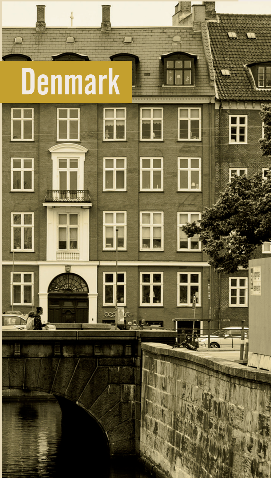
Storm bridge, Copenhagen
